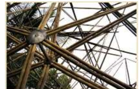
The metal joints at the nodes of the polygons
