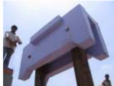
The wooden joint at the junction of column & beam
