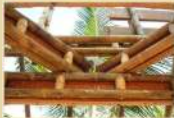
Primary & secondary beams
