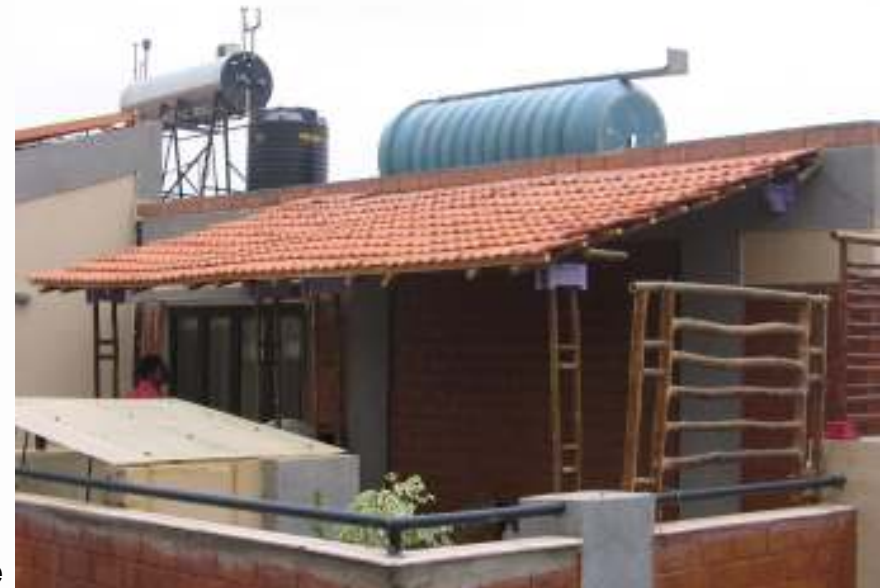
The finished structure
