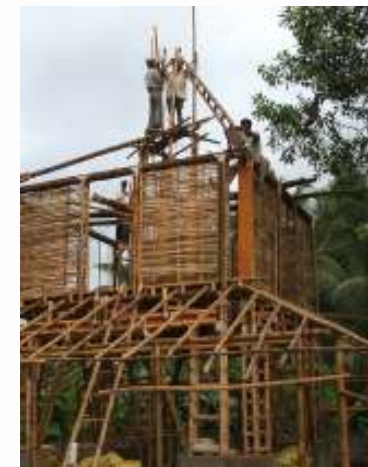
Principal rafters of the roof being placed
