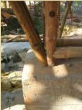
Column-beam Junction
