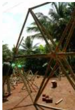
Hexagonal and pentagonal components being fabricated
