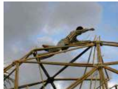
Polygonal components being assembled
