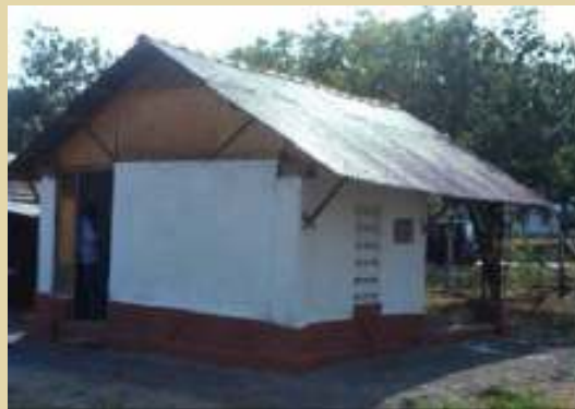
A finished dwelling unit
